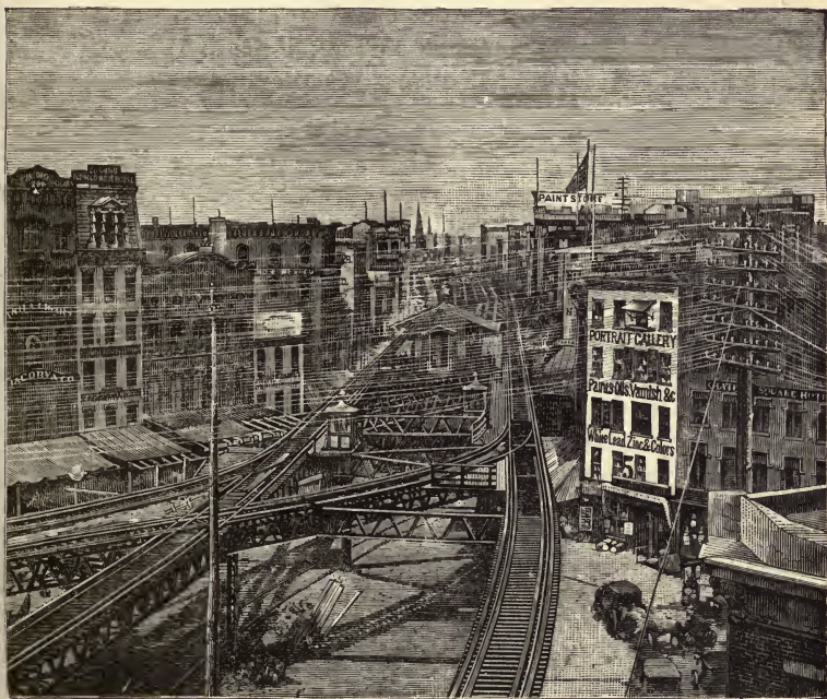
THE ELEVATED RAILWAY. • View in Chatham-street.
